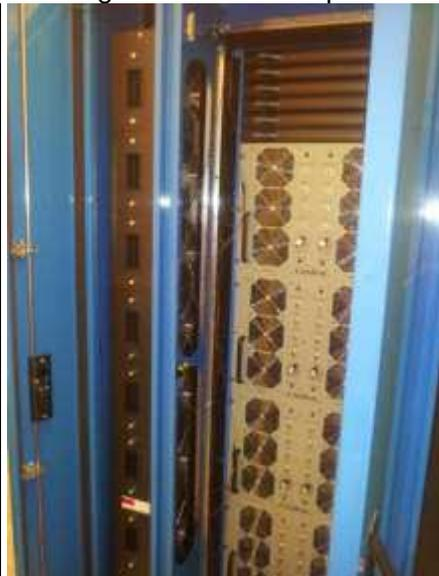
R.A.S.E.R. HD additional sensors, load-banks and one exchanger
